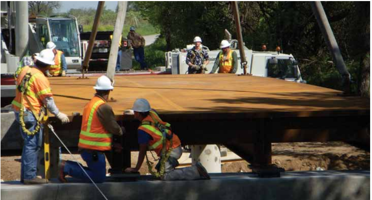
Installation of new SPS Bridge Deck
