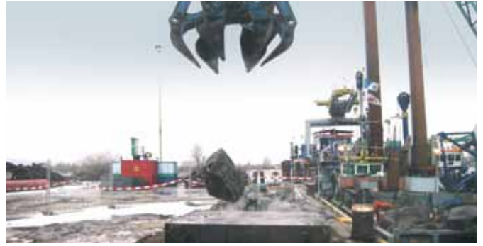
SPS impact test dropping 2 tonne rocks from 3 metres onto a section of SPS deck. SPS sustained no damage; the all-steel equivalent was destroyed.
